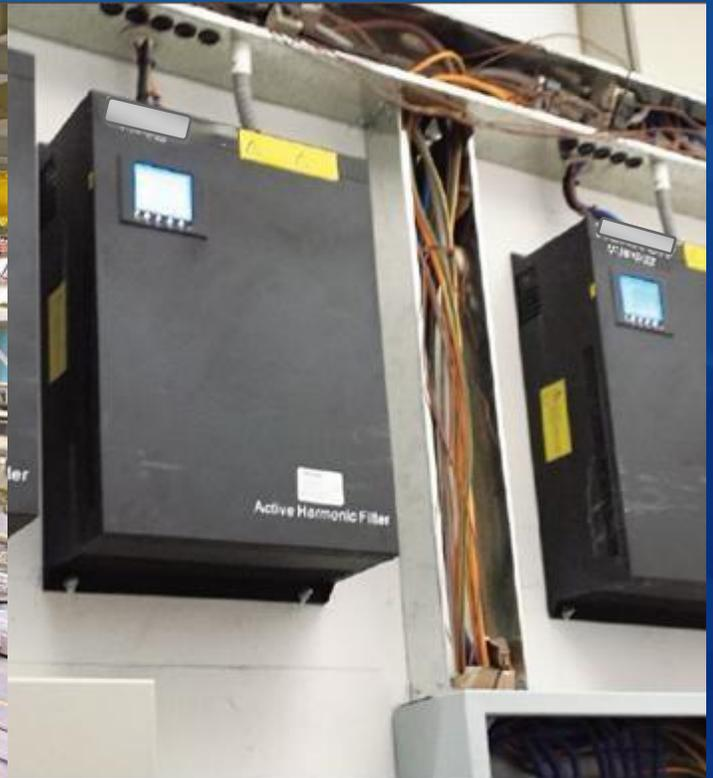
After the source filter is turned on, the waveforms are close to the standard sine wave, especially the current waveform, which is compensated from the very distorted waveform to a relatively regular sine wave. The number of times is mainly 5th, 7th, 11th, 13th, 17th, and 19th. After compensation, the harmonic current content is significantly reduced to achieve a perfect compensation effect.
