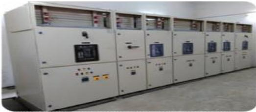
**ACB Panel for Power distribution and Control up to 6000A**
